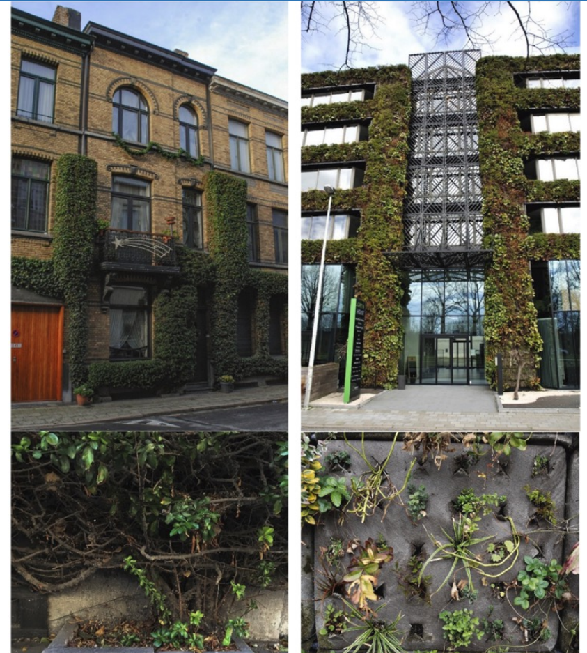
Fig. 1. On the left a direct green façade (GF) and on the right an living wall system (LWS) placed in a city. Below these pictures, the rooting system of the GF and the support structure (here a panel made of rockwool) of the LWS. (Ysebaert et al. 2021)
